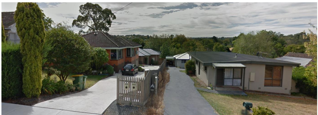
Photograph 16: Looking toward 2-lot developments at No. 12 & 14 Central Avenue
