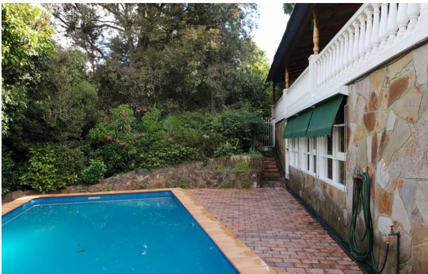
Photograph 8 : Looking across the rear of the dwelling
