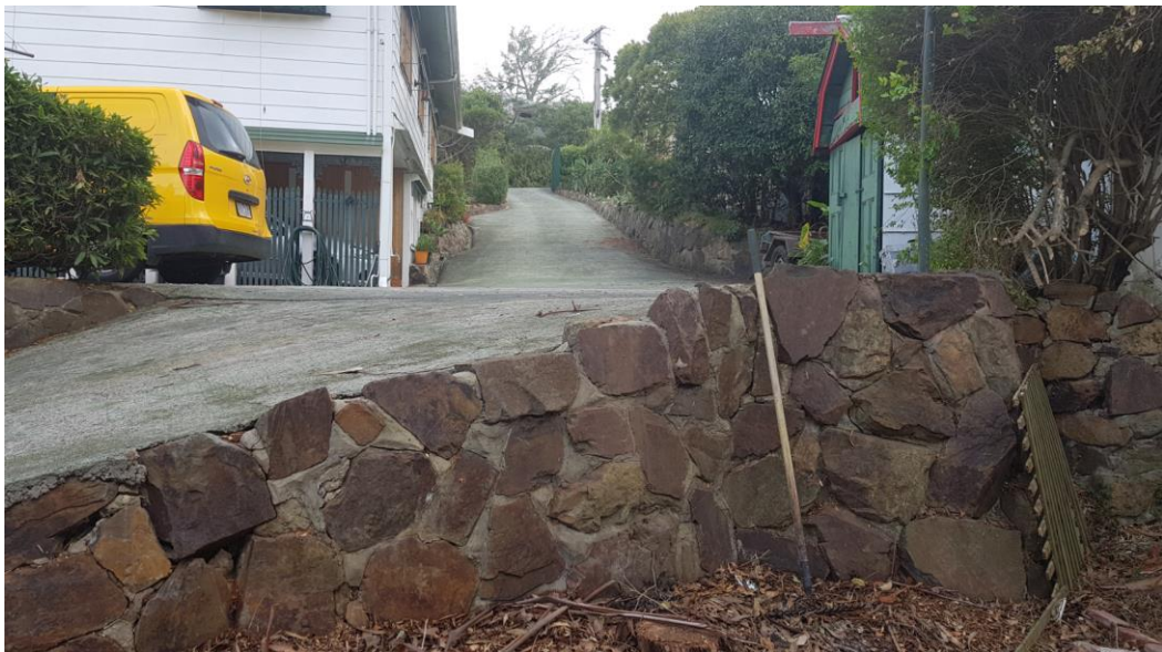
Photograph 5 : Looking south-west along the northern boundary and driveway
